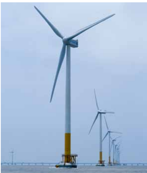
Figure 12 Panorama of the Donghai Bridge Wind Power Project
