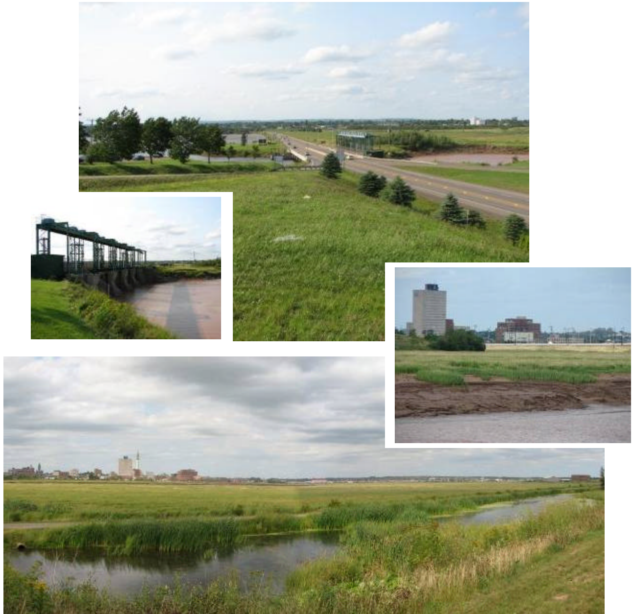
The road causeway over the R Pedicodiac at Moncton has led to significant build up of mud flat & salt marsh
