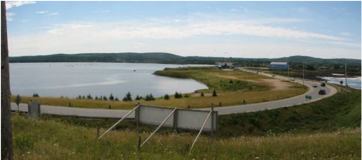
The causeway across the R. Annapolis with the tidal power plant; upstream to the left and downstream to the right.
