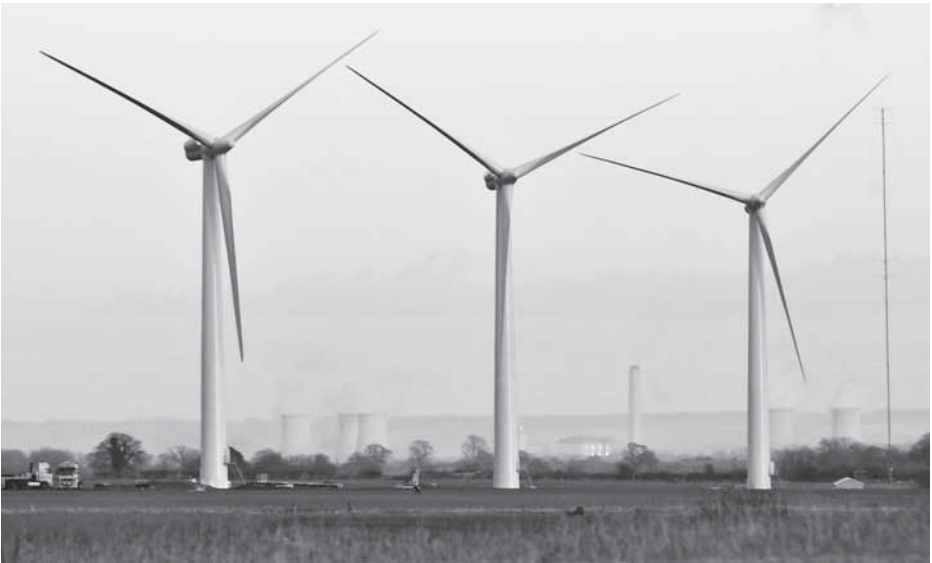
Figure 9 Construction of the Westmill wind farm, Oxfordshire, England. Photo by Martin Phelps of Westmill Wind Farm Co-operative.
