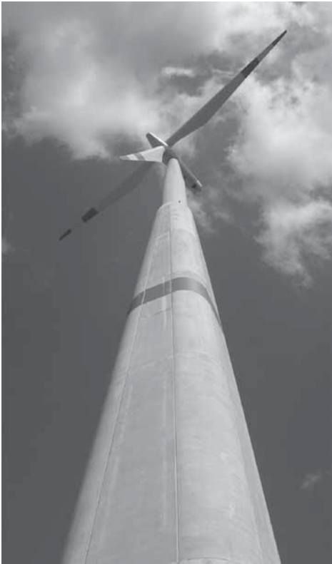
Figure 4 ATS Hybrid tower. Photo: ATS.
