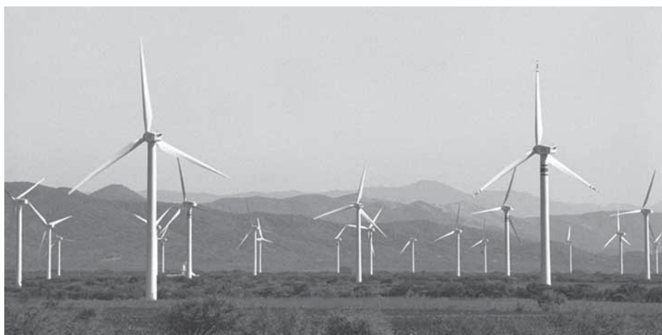
Figure 2 La Venta II 83.3-MW windfarm on the Isthmus of Tehuantepec, Mexico.
