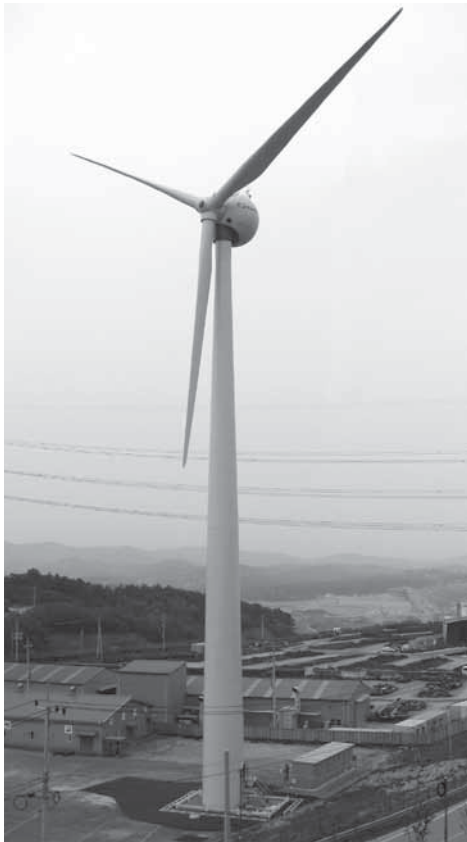
Figure 1 Unison's first commercial product of 750-kW direct drive, U50, has been installed in Korea Hydro & Nuclear Power Co., Ltd.
