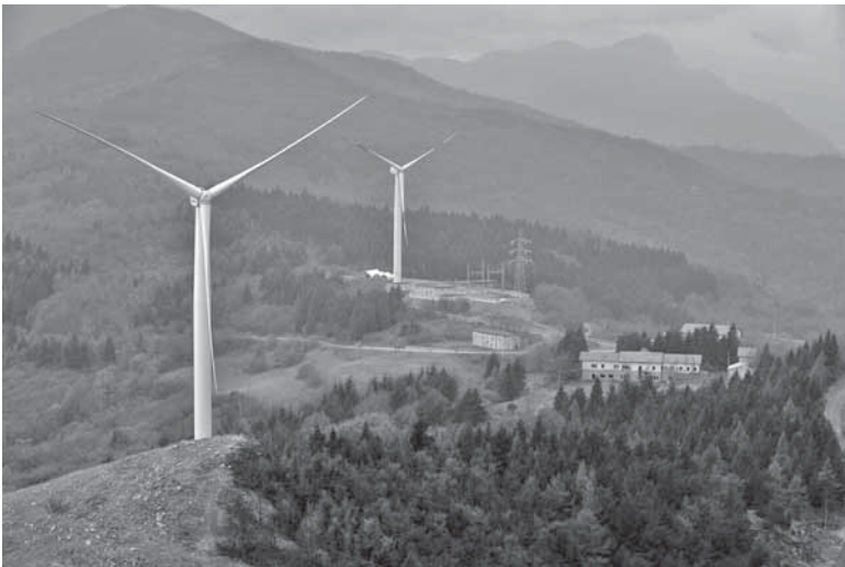
Figure 8 Nordex 2.5-MW NM 90 turbines at Garessio (Cuneo) in the Italian Alps (courtesy of Nordex Italia).
