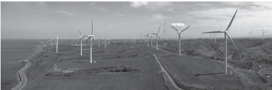
Figure 5 A view of Tomamae wind farm region.
