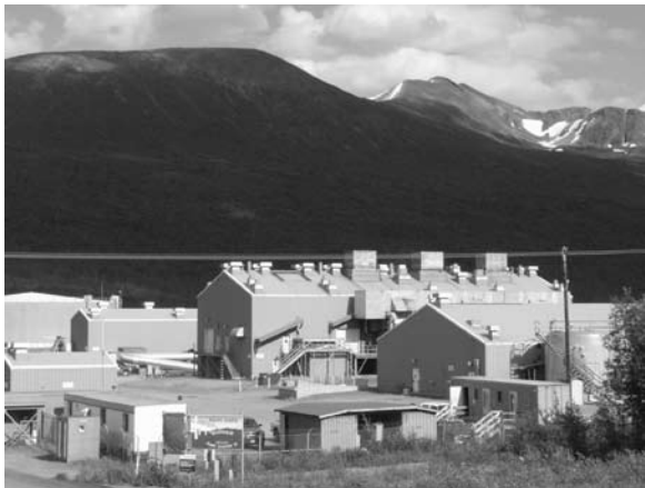
Pump Station 12, 65 miles north of Valdez, is in the southernmost station, pushing the oil up and over Thompson Pass.
