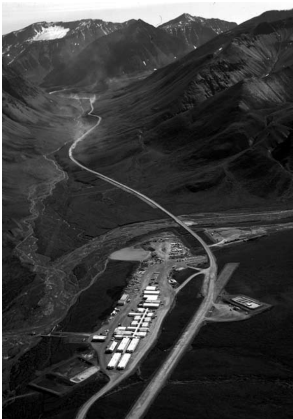
Atigun Construction Camp was one of 30 camps operating during pipeline construction. The buildings were removed and the site was revegetated in 1978.
