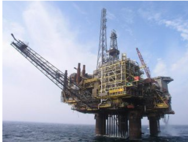
Exhibit 8-3. An offshore structure supported on concrete pilings.
