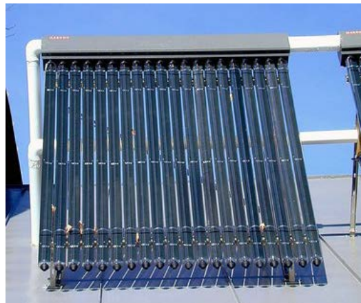
Figure 3. Evacuated tube collector
