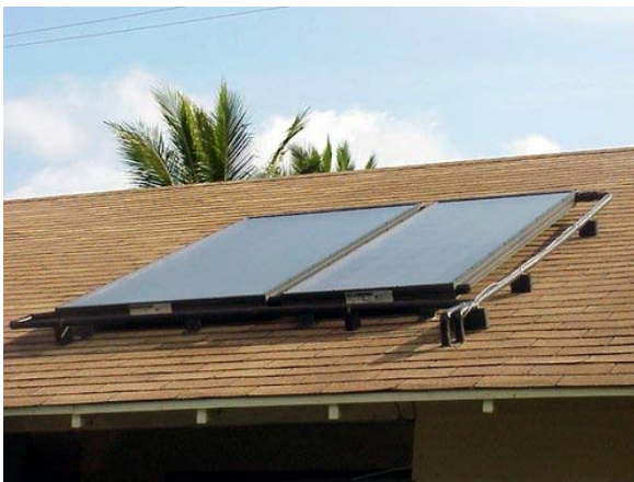
Figure 2. Flat-plate collector
