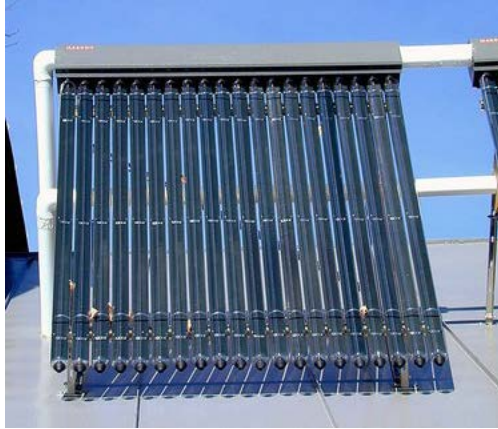
Figure A–2. Evacuated tube collector. Photo by Alan Ford, NREL/PIX 09501
