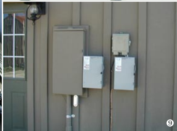
(top) Photo courtesy of Decker Homes. (bottom) Photo courtesy of Leif Juell, Alternative Power Enterprises, Inc.
