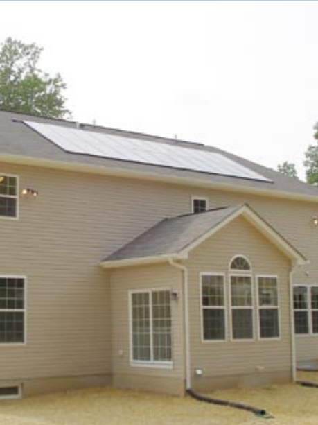
(left) The BP Integra PV system (above) hugs the roof line.
