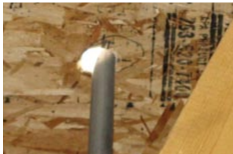
Photos courtesy of Namaste Solar Electric
