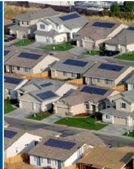
A view of the 95 homes of Premier Gardens, all today's zero energy. Photo courtesy of Sacramento Municipal Utility District.
