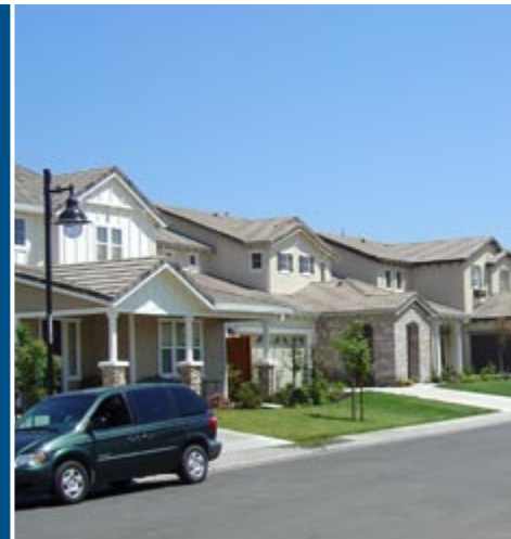
(above) It is difficult to pick out houses with integrated photovoltaic systems. All of these homes are so equipped.
