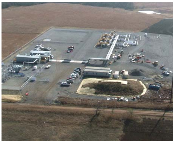
Figure ES-7 Pump Station on the Existing Keystone Oil Pipeline System
