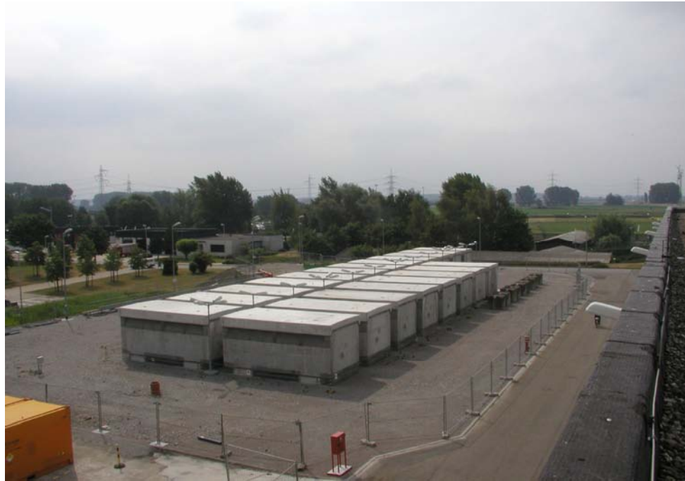
Figure 4. Interim storage area at Biblis NPP
