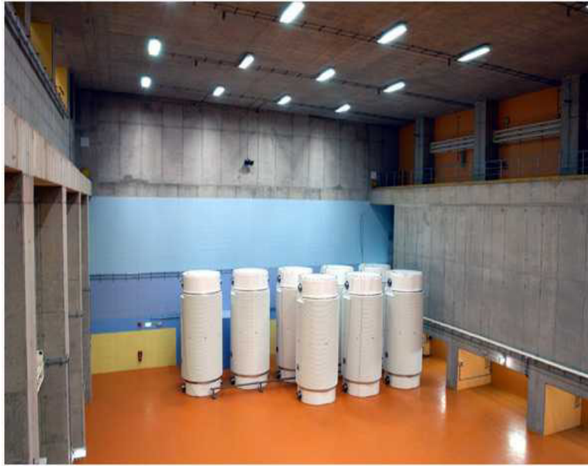
Figure 2. Interim storage facility at Lingen NPP
