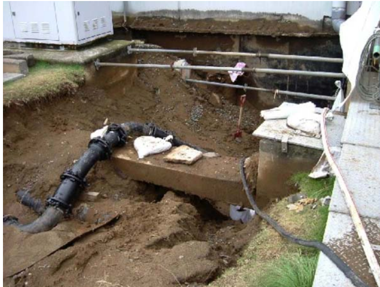
Figure 4-5 Failure of Underground Piping
