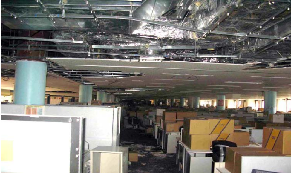
Figure 4-1 Ceiling Damage in Administration Building
