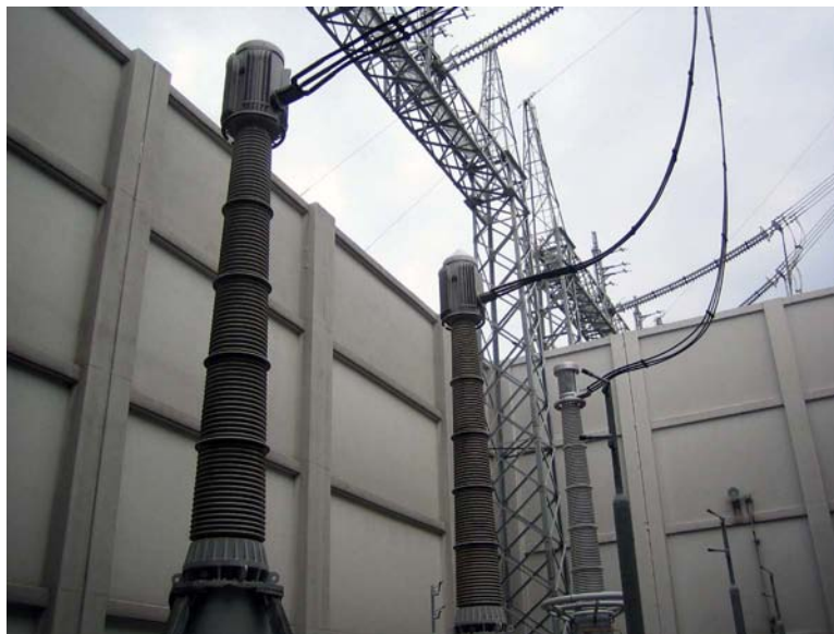
Figure 4-4 Bushing Plate Junction to Termination Stack
