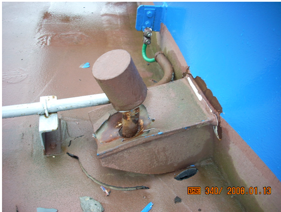
Figure 4-2 Damage to Domestic Water Tank Anchorage in KK Plant Yard
