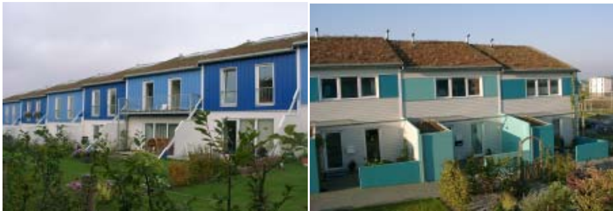
Figure 4: South and North views of the Passive House rows in Hannover-Kronsberg
