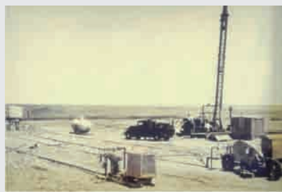
Fig. 1 —In 1947, Stanolind Oil conducted the first experimental fracturing in the Hugoton field located in southwestern Kansas. The treatment utilized napalm (gelled gasoline) and sand from the Arkansas River.
