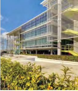
Abengoa headquarters, Seville, Spain / Credit: Abengoa.com
