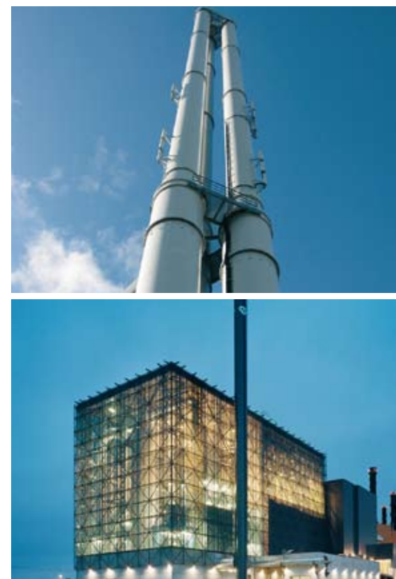
The Nordic countries extract the most energy from waste through incineration. Sweden recovers more than any other country. The pictures show the incineration plant in Trondheim, Norway, and Gärstadverket in Linköping (bottom picture) Photo: Åke E:son Lindman.
