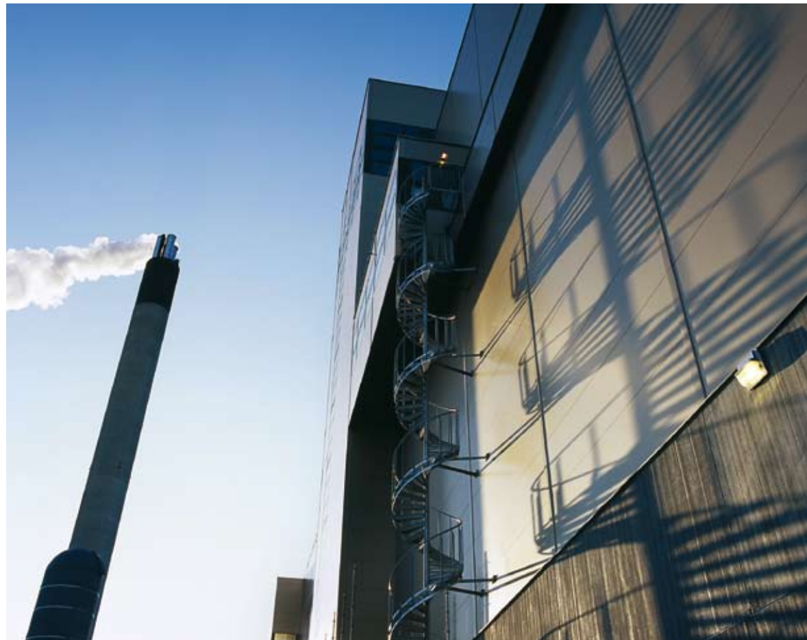
In 2006, the combined heat and power (CHP) plant for waste fuel at Korstaverket in Sundsvall became operational. Photo: Torbjörn Bergkvist
