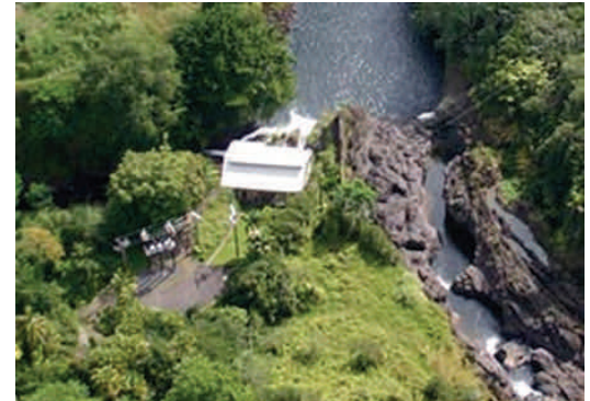
1.1-MW Waiau Hydro Power Plant on the Wailuku River, Hilo
