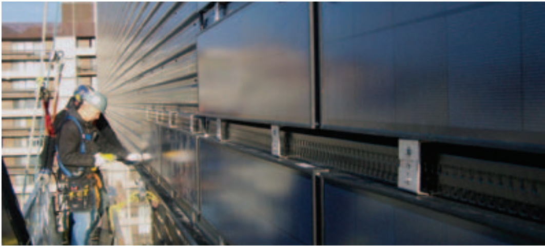
Photo 4.8 Installing a solar air heating system
