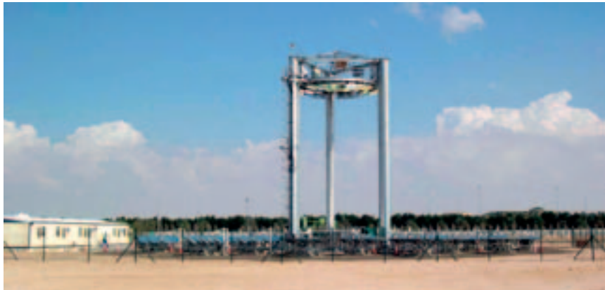
Photo 7.8 Experimental beam-down solar tower in Abu Dhabi
