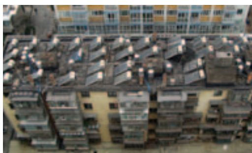
Photo 4.2 Solar water heaters in Kunming, China
