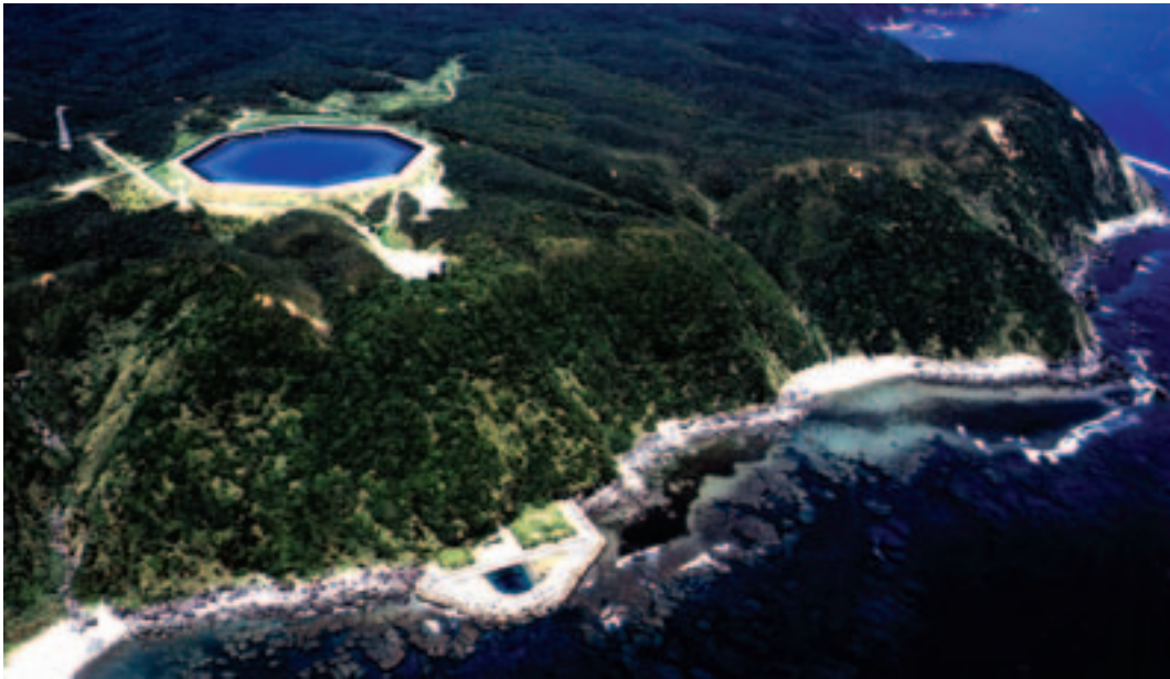
Photo 11.1 Okinawa's pumped-hydro plant using the ocean as lower reservoir
