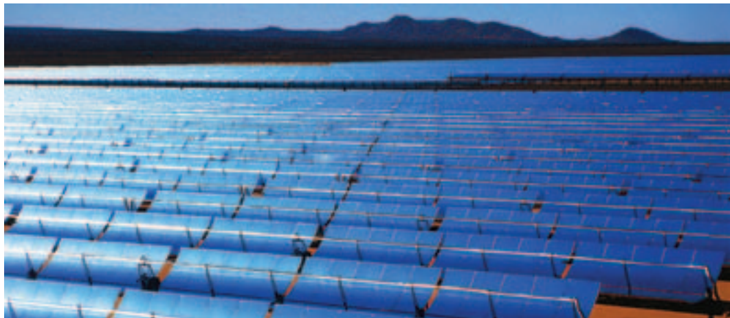
Photo 8.7 Partial view of the solar field of a CSP plant
