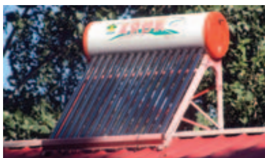
Photo 4.1 Chinese thermo-siphon solar water heater
