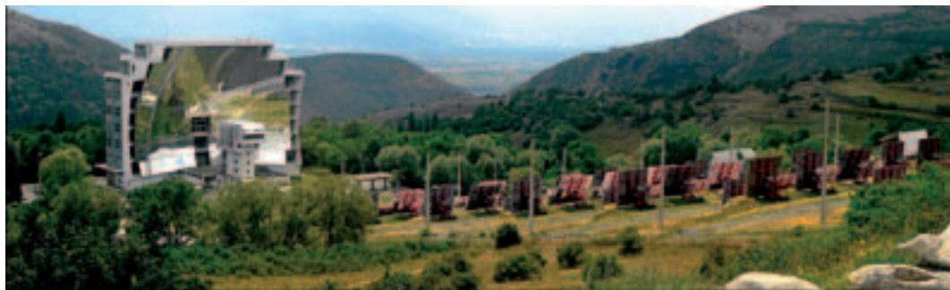
Photo 7.5 The solar oven at Odeillo (France)
