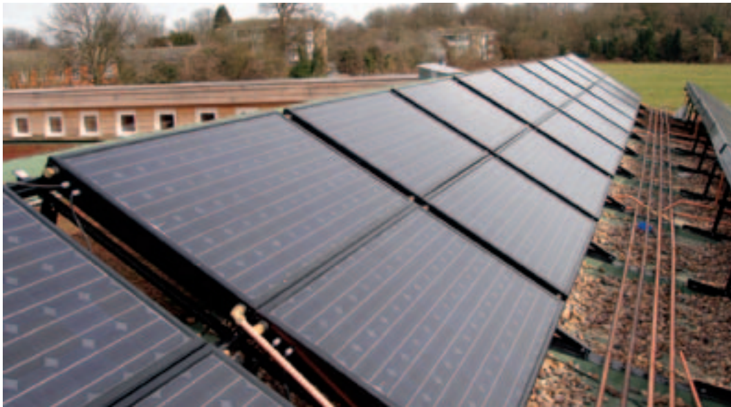
Photo 6.1 PV-thermal collectors manufactured in Turkey
