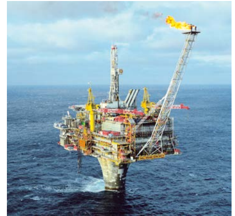
Oil Platform Draugen.
