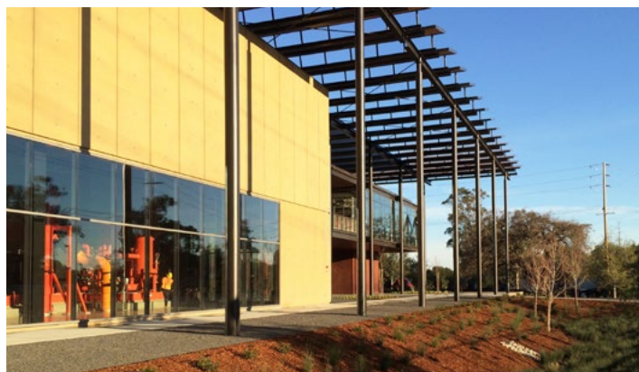
Photos: The Central Energy Facility
