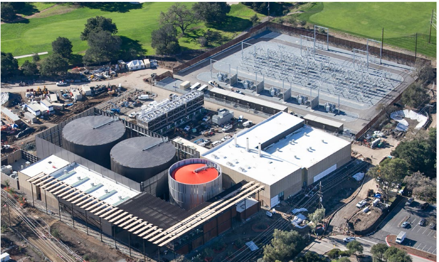
Photo: SESI represents a transformation of university energy supply from 100 percent fossil-fuel-based combined heat and power plant to grid-sourced electricity and a more efficient electric heat recovery system
