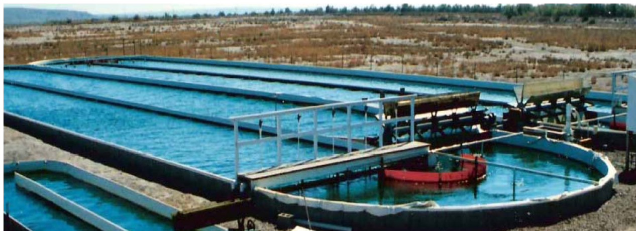
Figure 3.4: The Roswell Algae Test Facility, New Mexico (Weissman et al., 1988).
