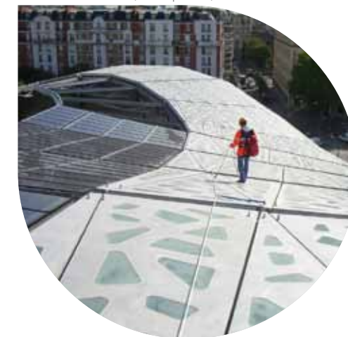
Jean Bouin Stadium, solar panels, 16 th
