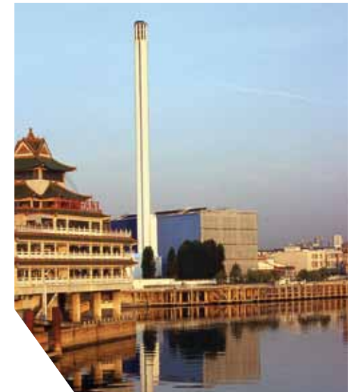
Heat production factory, Ivry-sur-Seine
