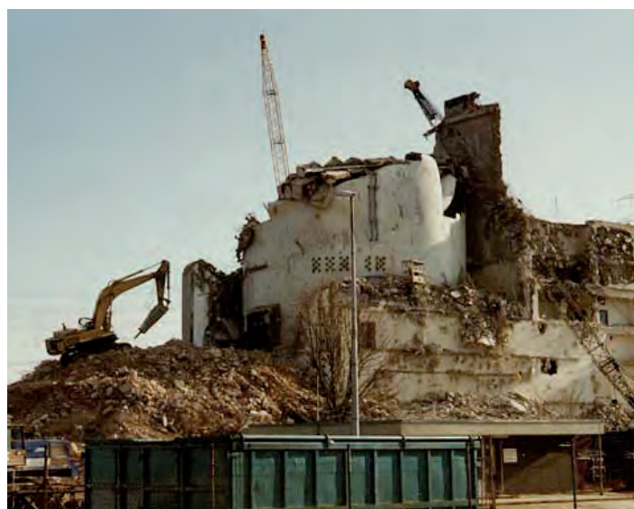
Fig. 17: Conventional demolition of the outer building shell of the Niederaichbach nuclear power plant
