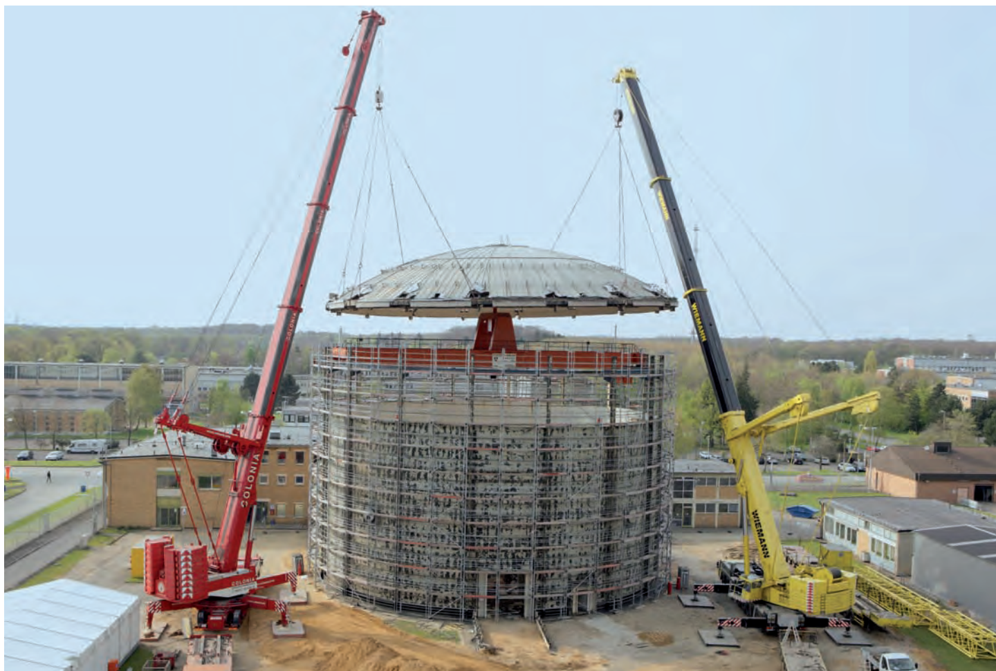
Fig. 6: Dismantling of the FRJ-1 research reactor
