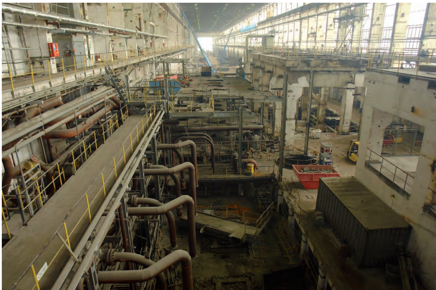
Fig. 41: Turbine building of the Greifswald nuclear power plant after removal of the generators
