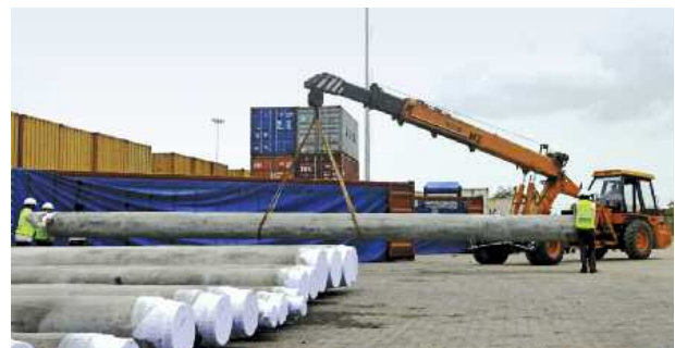
The first batch of cooling water piping reached ITER from India in 2015.
