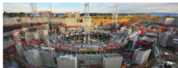
The first 200-degree segment of the ITER bioshield (inner circle, light grey) is poured in October.
