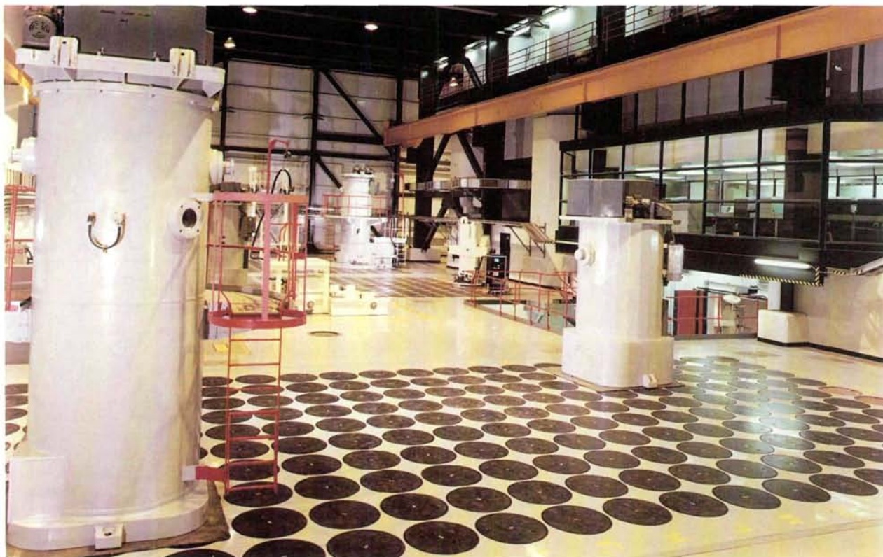
Storage of vitrified high-level waste. (Credit: BNFL)
