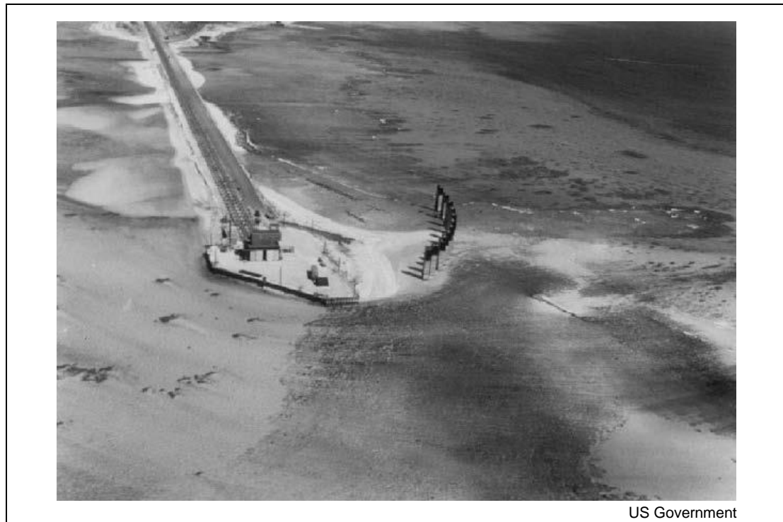
Figure 1-12. BRAVO shot site showing the causeway with vacuum line-of-sight pipes connected to the shot cab
