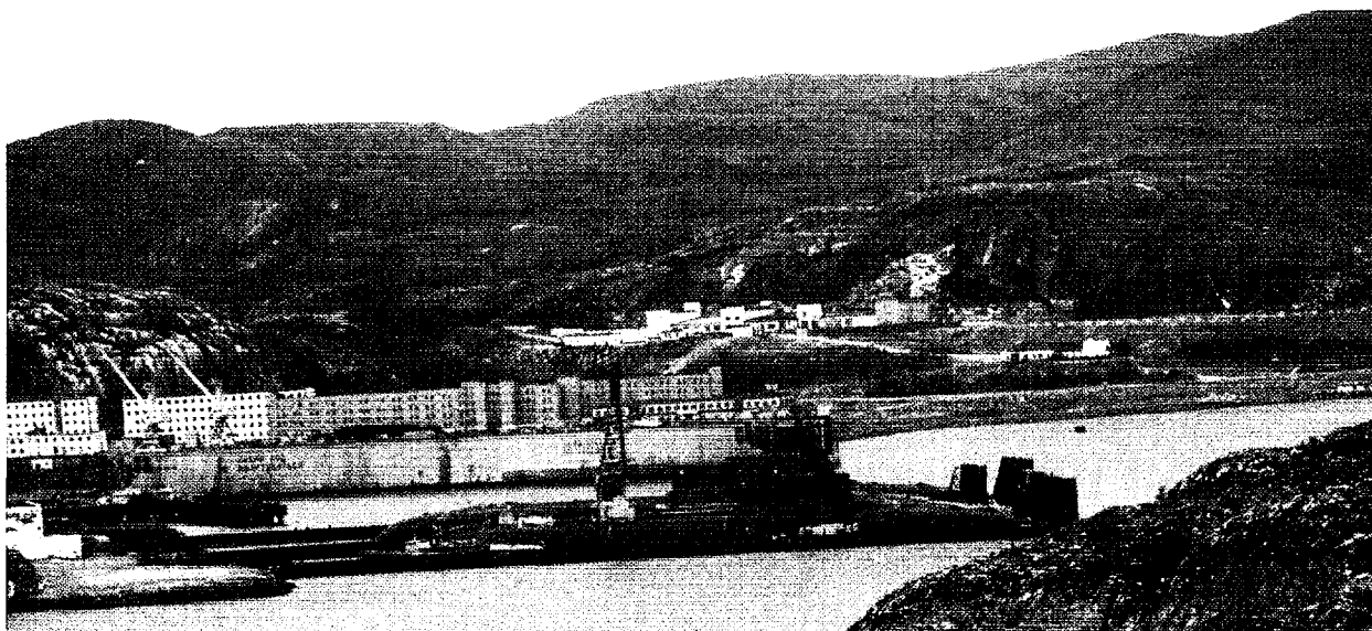
Nerpichya lies in the innermost reaches of the Litsa Fjord. The base facility also has a dry dock which is used for carrying out repairs on the Typhoon class submarines. There is also a smaller, temporary storage area for solid and liquid radioactive waste.
