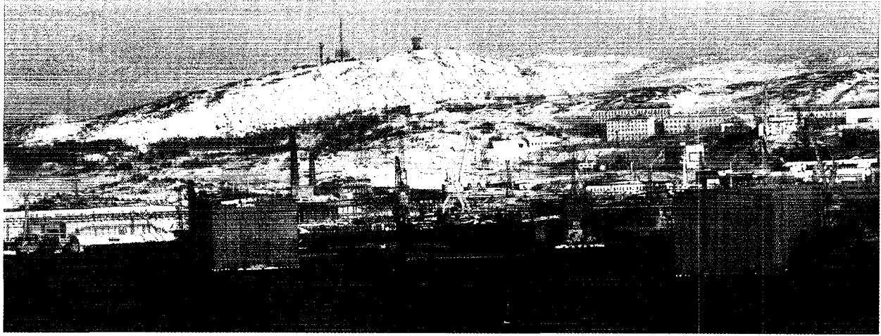
The naval yard Shkval lies close to the city of Polyarny, and it is here that maintenance work on the laid up submarines is carried out as well as the servicing of second and third generation nuclear submarines that remain in service. The shipyard has a larger storage facility for solid radioactive waste and two floating tanks containing liquid radioactive waste. The nuclear submarine K-192 is also moored here with its melted down nuclear reactor following an accident in 1989.
