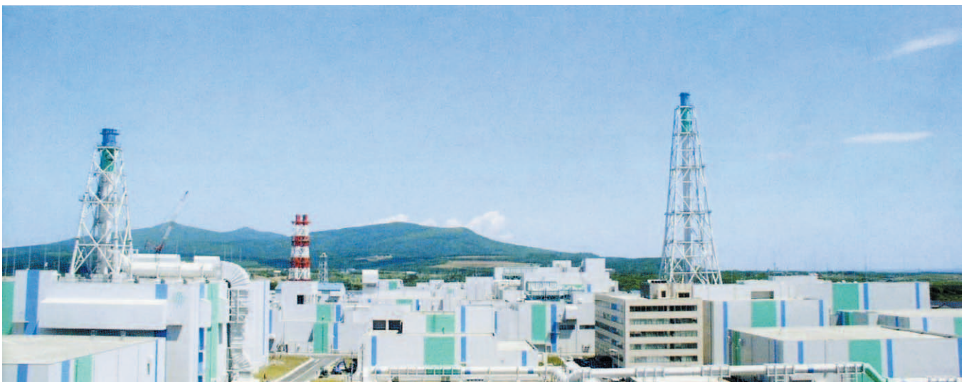
● Rokkasho Reprocessing Plant
