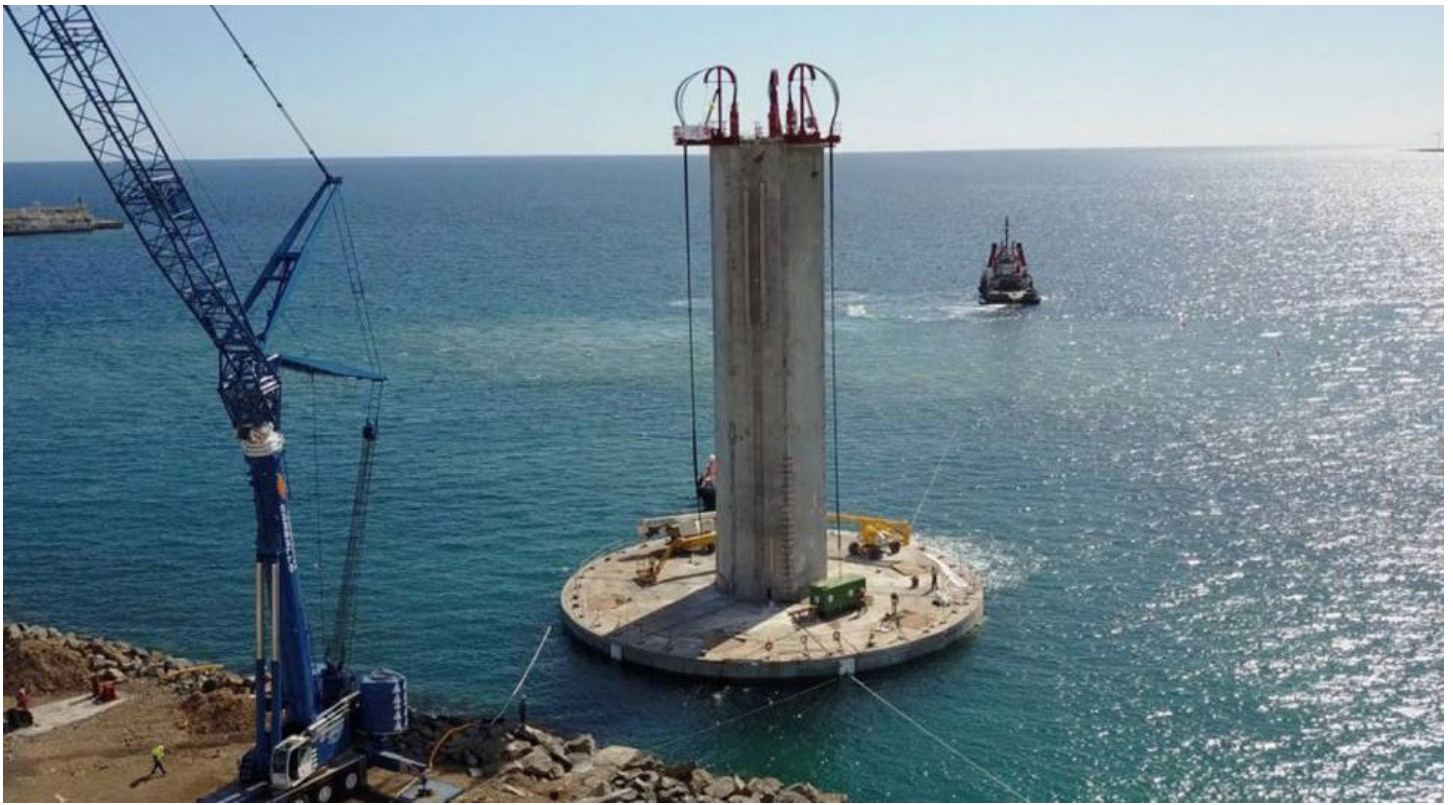
Figure 3. ELISA-ELICAN Project. 5-MW offshore wind turbine installed in Gran Canaria Island (Spain). Based on foundation gravity and with a telescopic tower, it is built of concrete and can be installed without the help of crane ships. (Photo credit: ESTEYCO)
