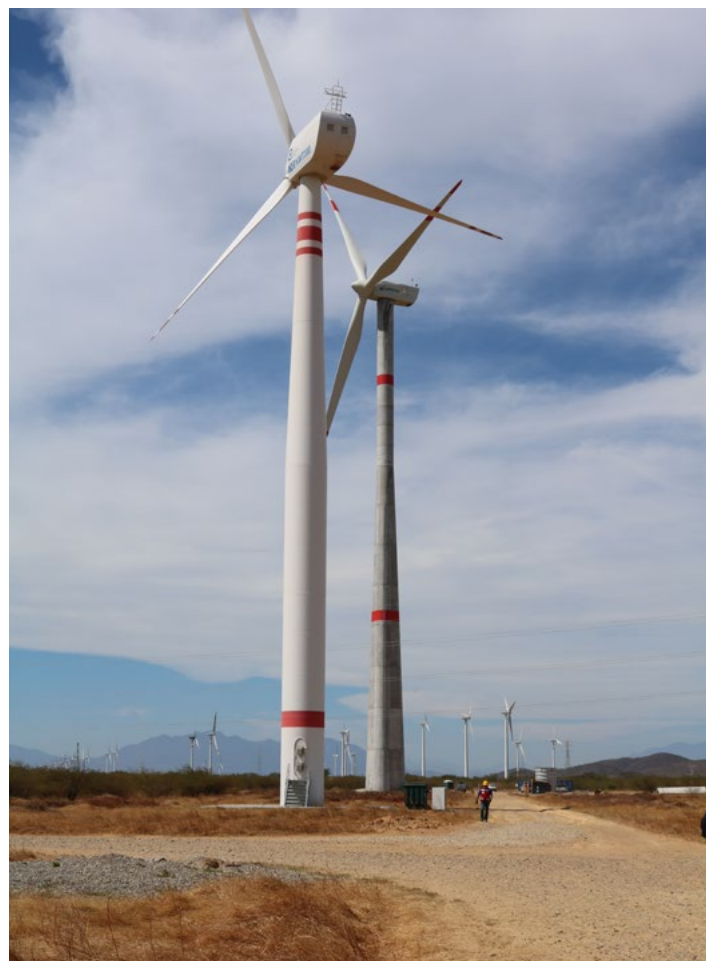
Figure 3. The Regional Center for Wind Technology (CERTE) in Oaxaca, México (Photo credit: © INEEL)
