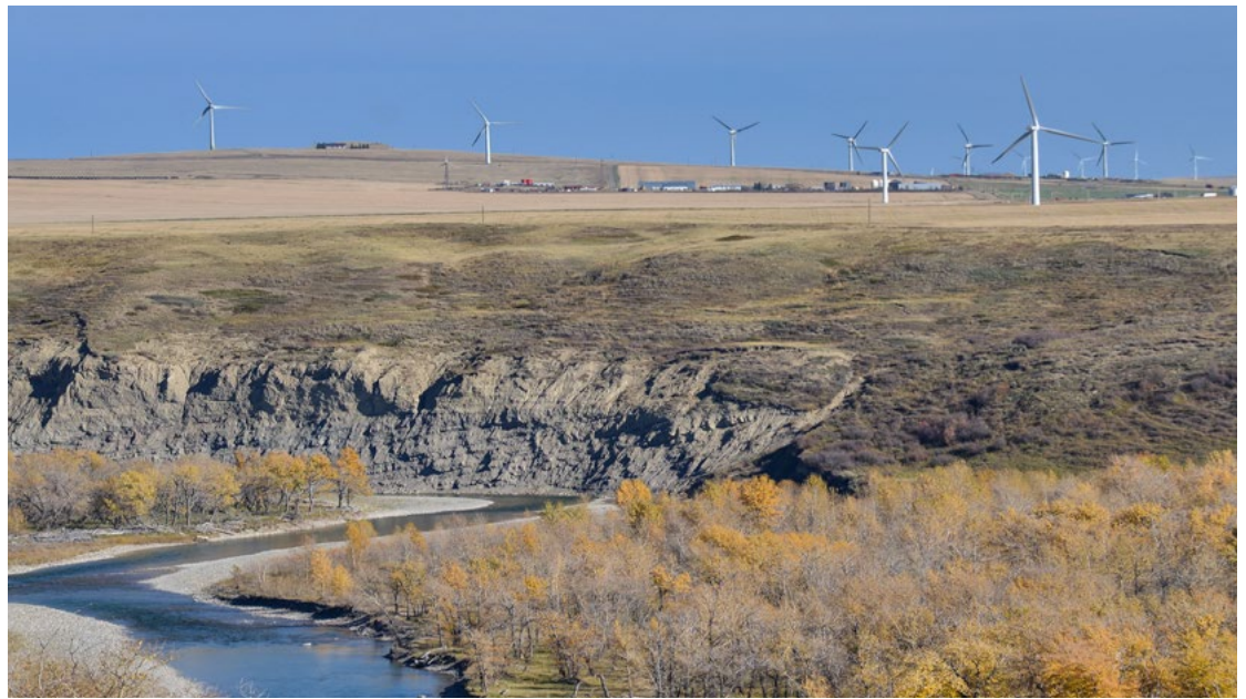
Figure 2. Castle River Wind Farm, Alberta featuring Vestas V47 turbines (Photo credit: Canadian Wind Energy Association (CanWEA)/Bryan Passifiume)
