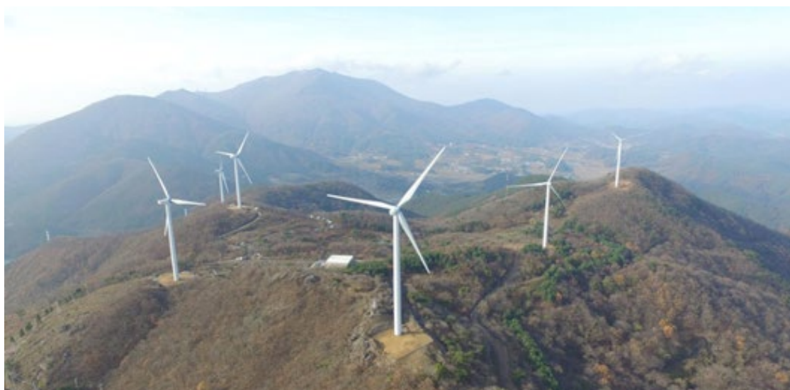
Figure 3. Hwasun Wind Farm, Republic of Korea (Source: Unison Co., LTD)
