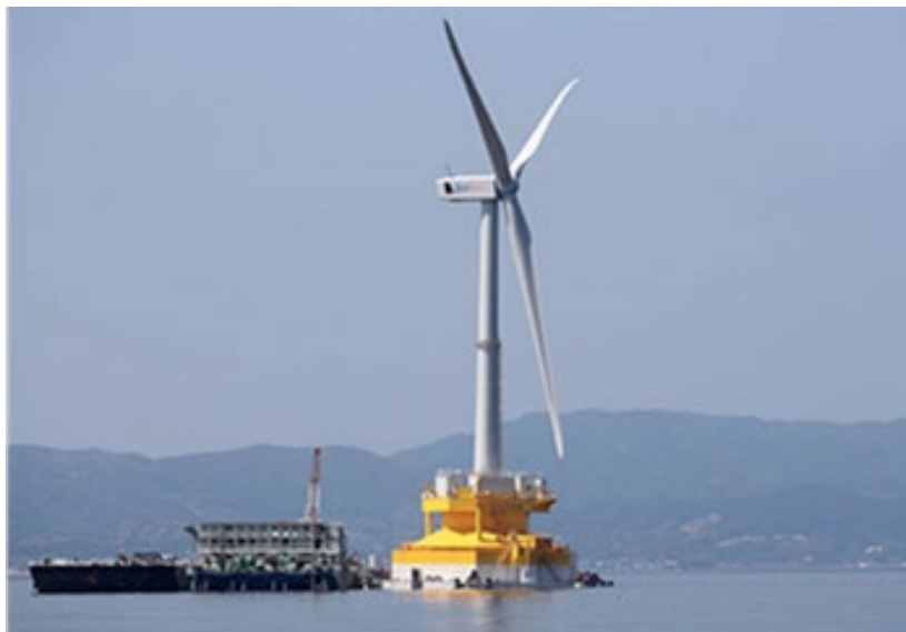
Figure 3. Hitachi 5-MW floating offshore wind turbine (Fukushima FORWARD)
