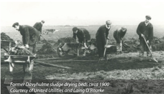
Pumping station under construction Courtesy of United Utilities and Laing O'Rourke
