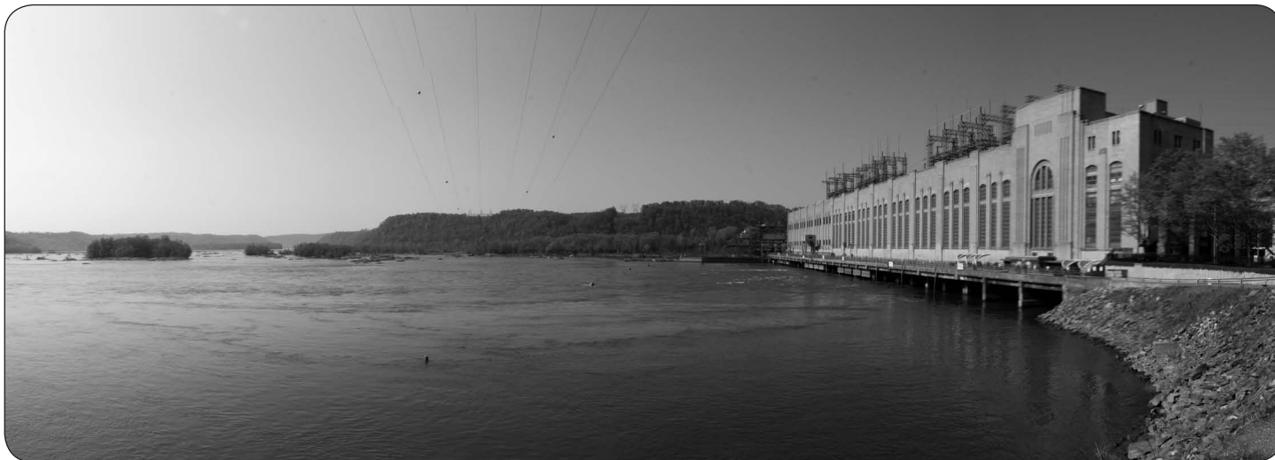
The down river side of a hydropower plant on the Susquehanna River in southern Pennsylvania.
