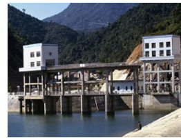
Guangzhou Pumped Storage Power Station
