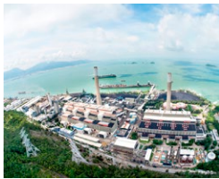
Castle Peak Power Station
