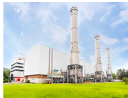
Penny's Bay Power Station
