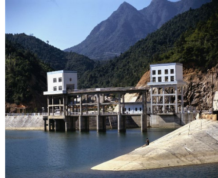
Guangzhou Pumped Storage Power Station, Guangdong
