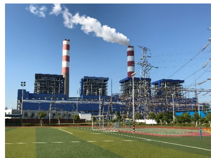
Fangchenggang I & II Coal-fired Power Station, Guangxi
