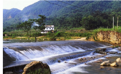
Huajji Hydro Power Station, Guangdong
