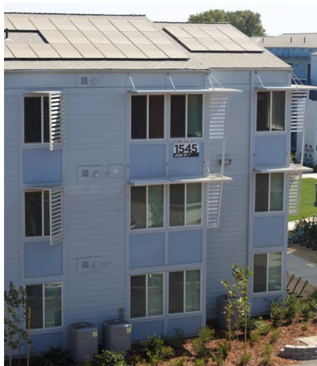
Figure 3. Ramble A style apartment building showing exterior window sunshades, rooftop solar photovoltaics (PV), and high efficiency heat pumps
