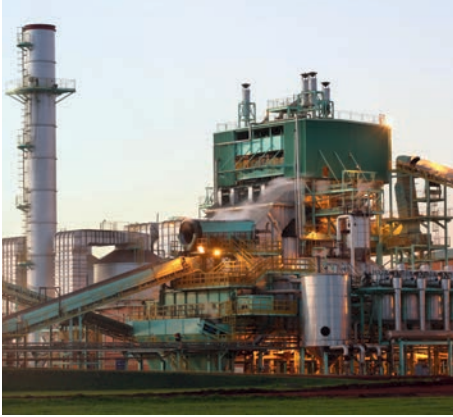
▲ Sugar cane reception, preparation and juice extraction facilities at BP Biofuels' Ituiutaba plant in Brazil.
