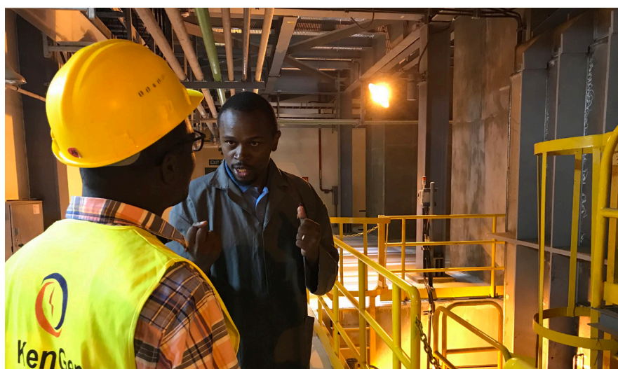
KenGen engineer explaining geothermal power generation at Olkaria IV © OLIVER JOHNSON
