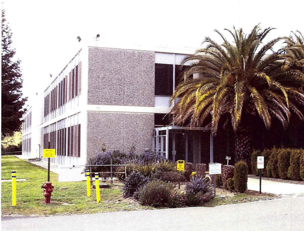
Photo 2.3 – Building 103 southeast corner view
