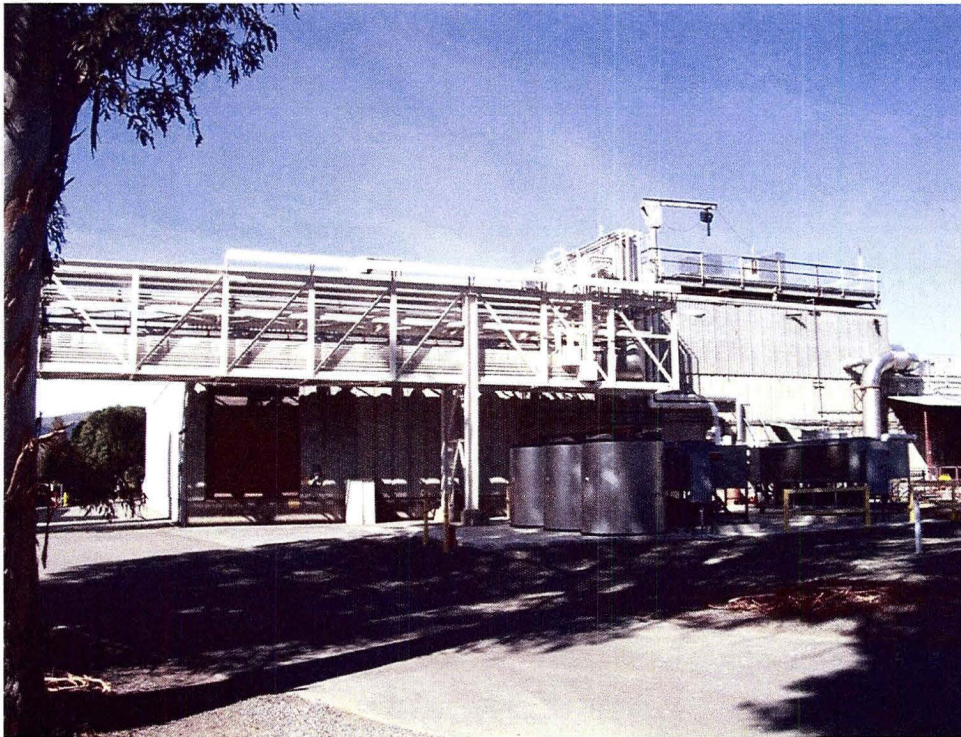
Photo 2.1 – Building 102 east side
