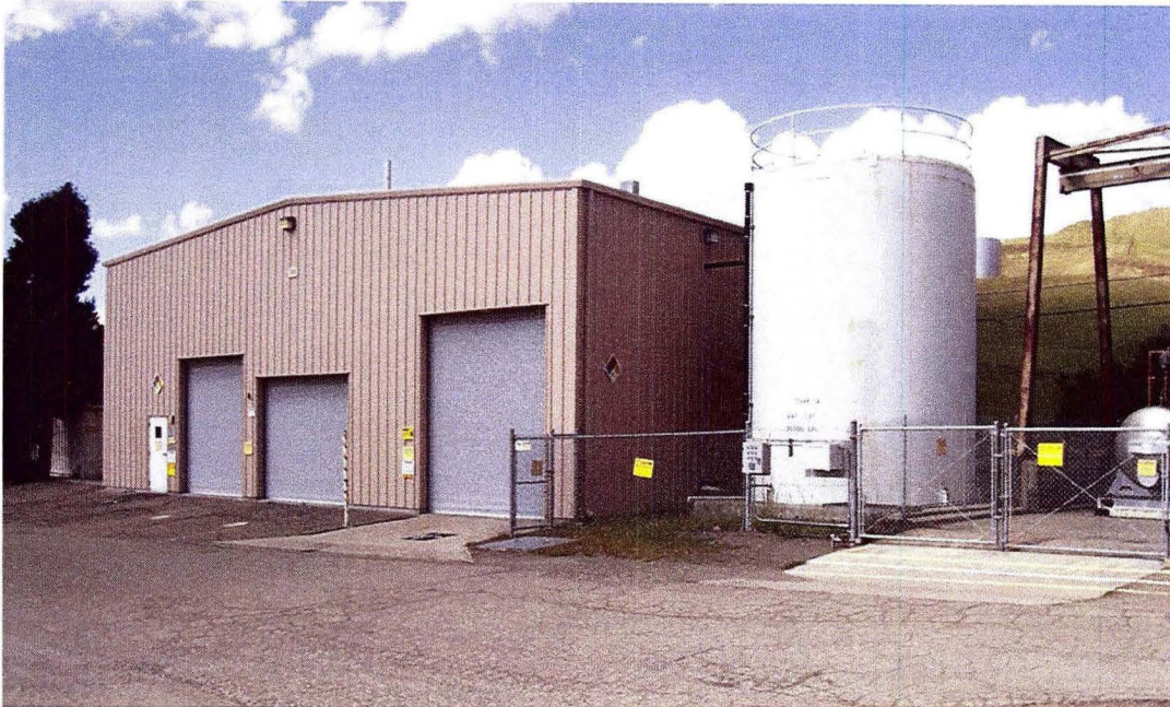
Photo 2.6 – WEP view of southside and 30,000 gallon tank
