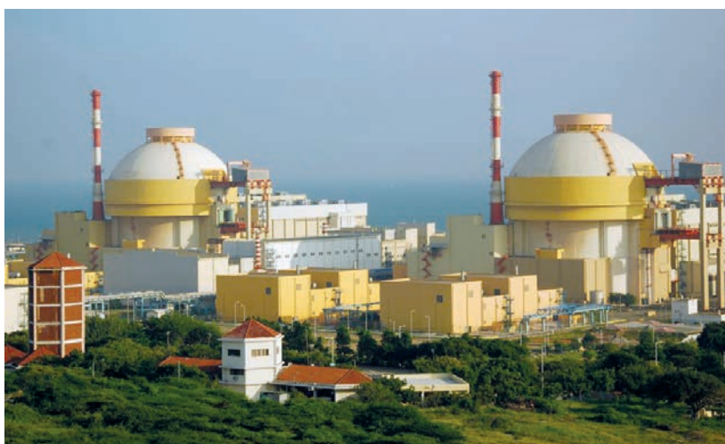
Kudankulam nuclear power plant
