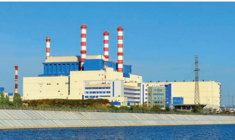
Unit 4 of the Beloyarsk plant: Image Rosenergoatom
