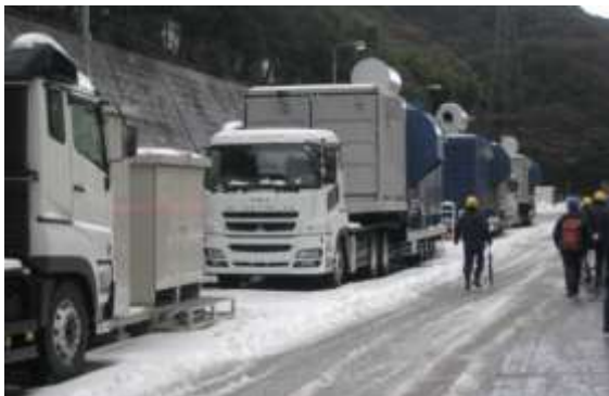
Place mobile units on a hill (mobile AC power source)
