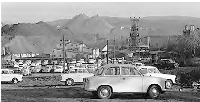
Figure 2.6. Parking lot and mine shafts at Schlema uranium mine with waste rock piles in background, 1965
