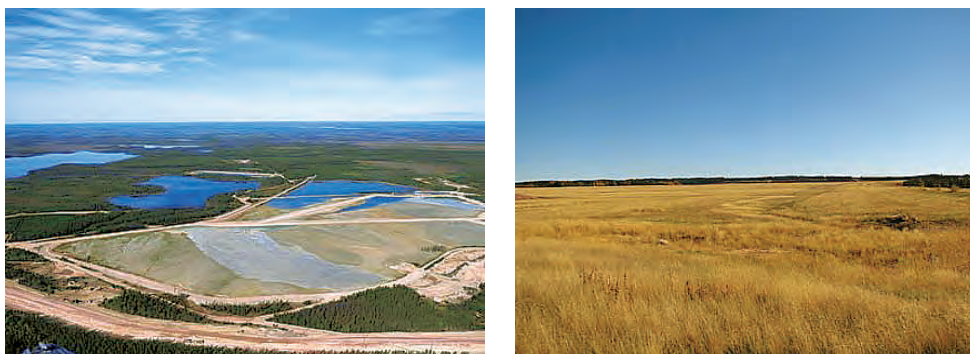
Figure 2.17. Cluff Lake TMA prior to decommissioning (left) and (right) after decommissioning and re-vegetation
