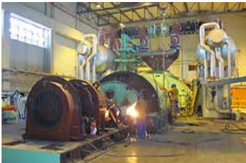
Figure 9.6: Dismantling of the turbine
