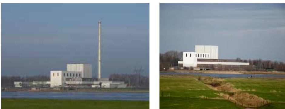
Figure 7.1: The Dodewaard nuclear power plant in operation (left) and in safe enclosure (right)
