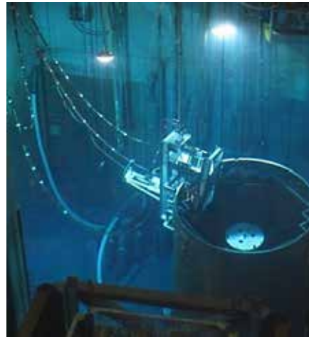
Figure 9.10: Segmentation of the lower internals
