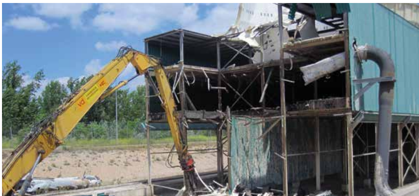
Figure 9.8: Demolition of cooling towers
