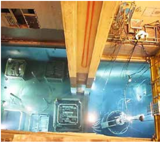
Figure 9.9: Reactor cavities during segmentation activities
