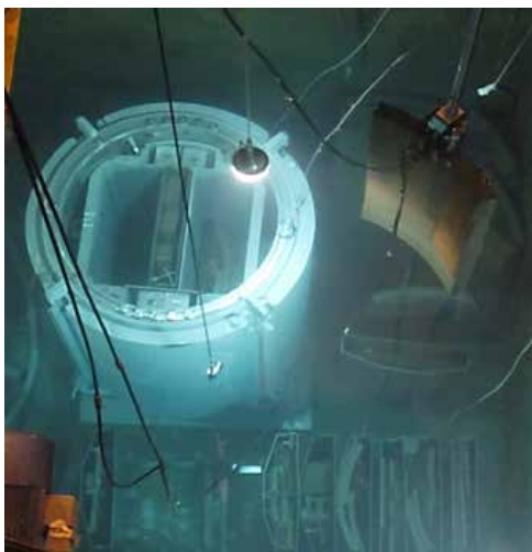
Figure 9.11: Special waste load containing the reactor internals
