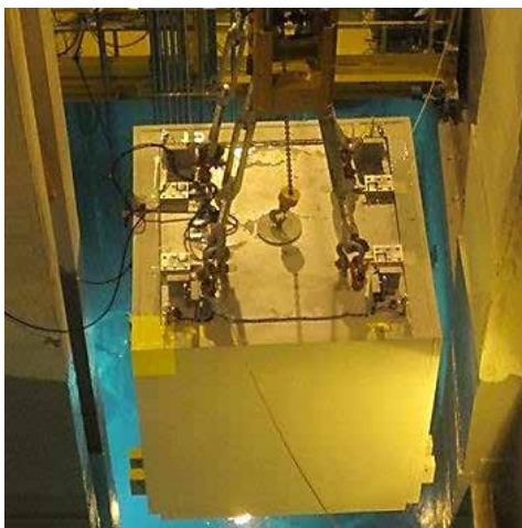
Figure 9.13: Removal of waste from reactor cavities for conditioning
