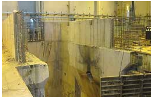
Figure 9.7: Works to reuse turbine building as radioactive waste storage
