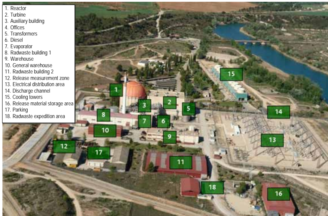
Figure 9.1: Site configuration during decommissioning projects
