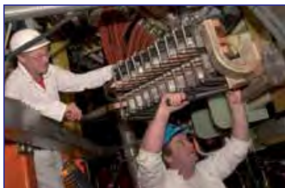
Figure 13: Maintenance work during 2004/2005 shutdown
