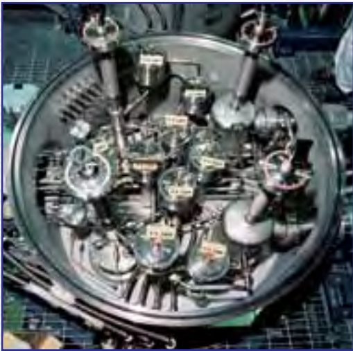
Figure 9: Module of the Cryogenic Forevacuum System (JET Active Gas Handling System)
