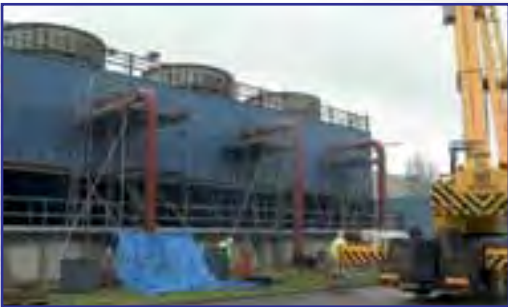
Figure 7: JET's cooling towers during major maintenance work in 2004
