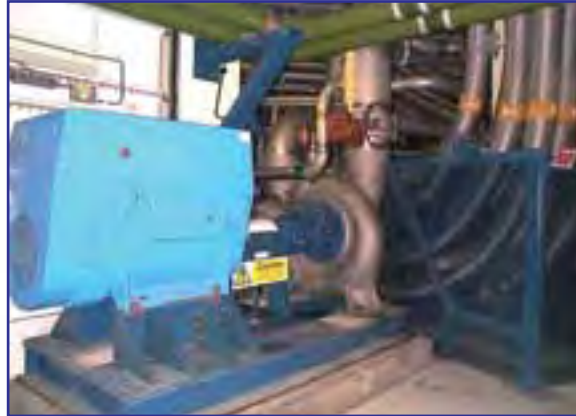
Figure 9: Neutral beam injector box cooling pump (in foreground) and the high voltage supply leads of the beam accelerators (in background)
