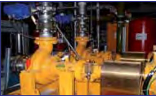
Figure 6: Poloidal field coils cooling pumps
