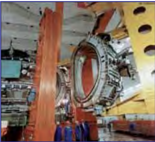
Figure 3: JET during construction (1982)
