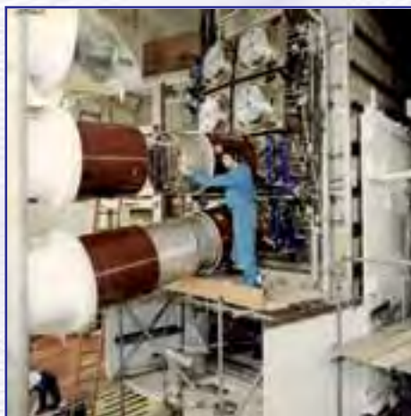
Figure 8: Installation of NBI at JET
