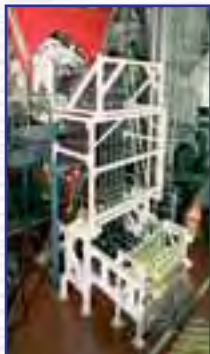
Figure 19: Connection of the LHCD waveguides to the JET vacuum vessel
