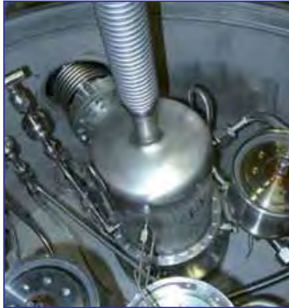
Figure 10: New pumping cryopanel installed
