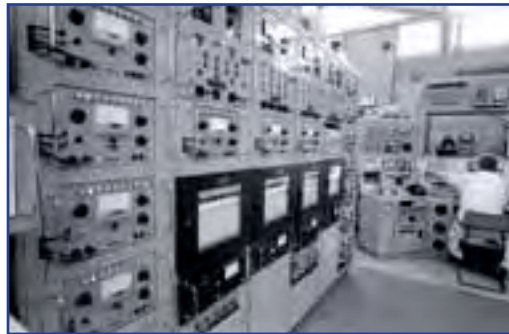
Figure 2: An experiment control room 40 years ago - lots of knobs and chart recorders
